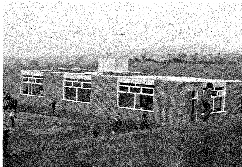
THE NEW ROMAN CATHOLIC SCHOOL, GLOUCESTER ROAD
